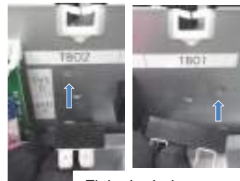
Fit in the hole
