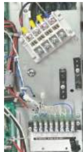
close-up view of terminal block sub-assembly
